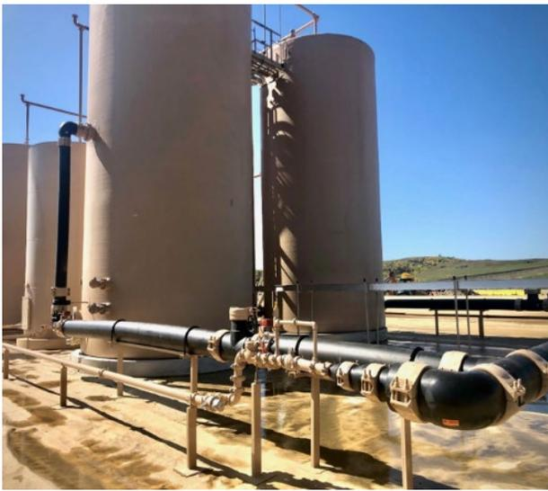
Permitted to accept up to 50,000 barrels per day (b/d) of produced water, the Crestwood Gondor Saltwater Disposal facility features two wells, two separators, two oil storage tanks, and 10 produced water storage tanks across nearly three acres. The project, which was constructed using both onsite installation and in shop fabrication, consisted of 12 inch and smaller HDPE pipe.
